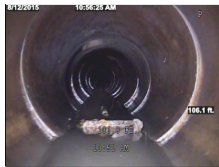
PICTURE 5 ASSUMED PIPE CONDITIONS
