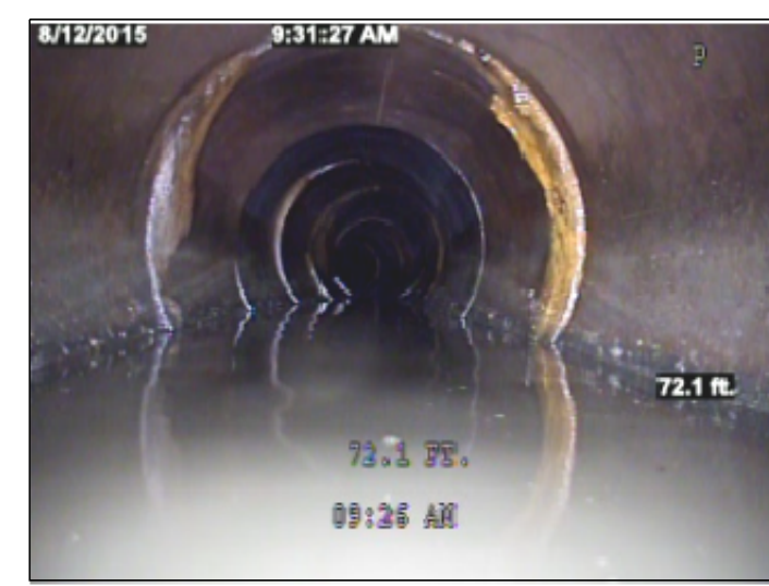
PICTURE 4 STANDING WATER IN PIPE
