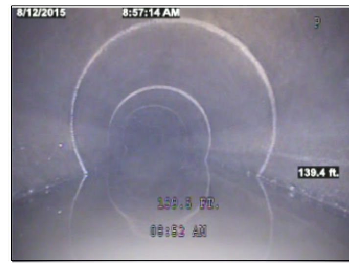
PICTURE 3 STANDING WATER IN PIPE
